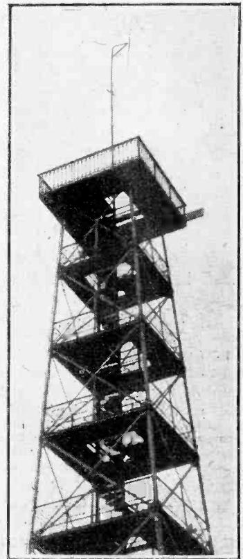
EXPERIMENTAL USW transmissions are being radiated from the top of the roof. observation tower of a hotel in Zürich, Switzerland. Above is seen the transmitting aerial, which has an effective height of 3,000ft. above sea level.
